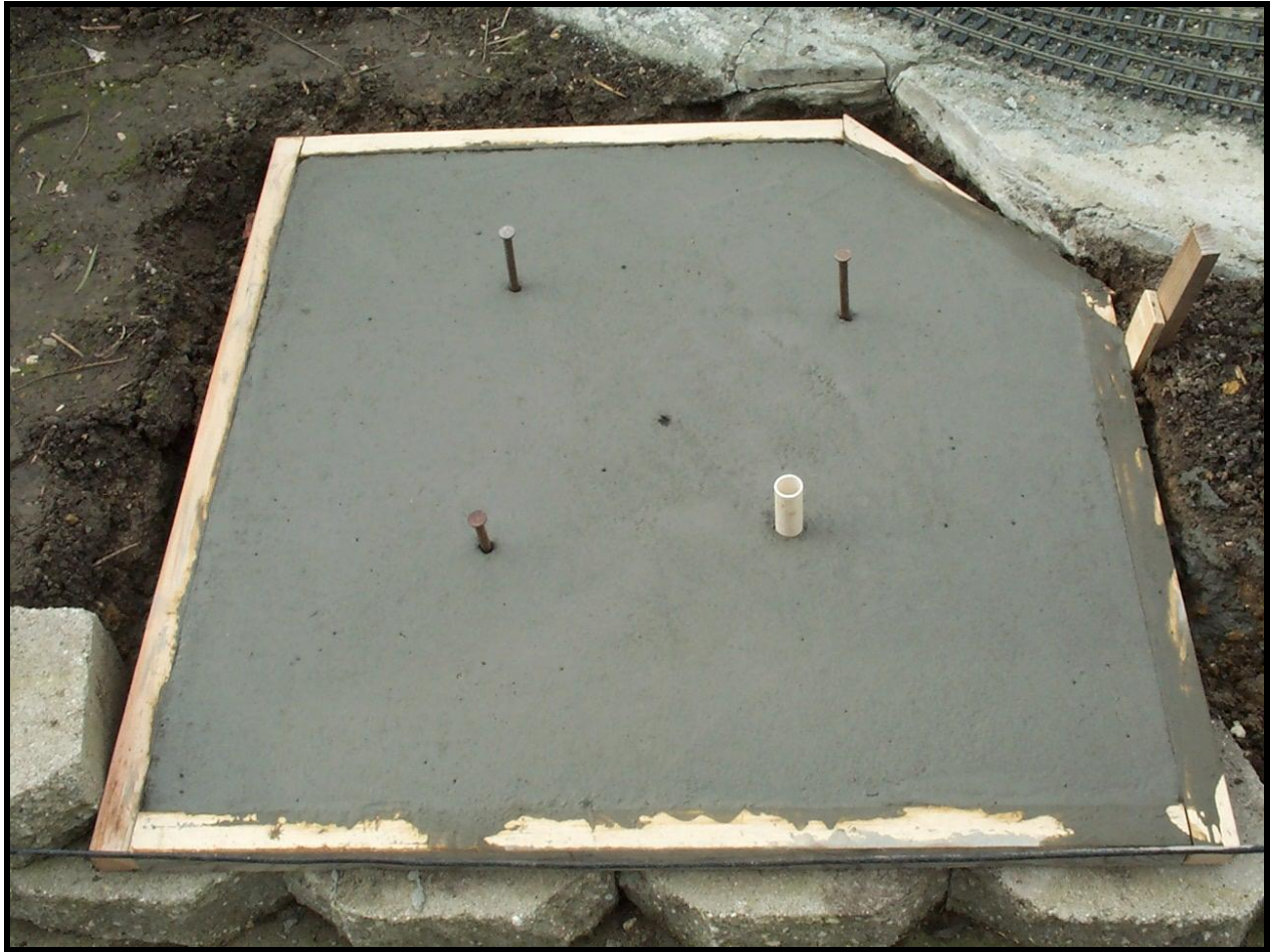
Pouring the turntable pad
